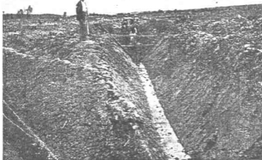
COCONUT ESTATE: DIGGING A FIVE-FOOT DRAIN.
