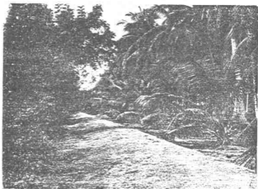
COCONUT ESTATE: A BUND TO KEEP OUT FLOOD WATER.
